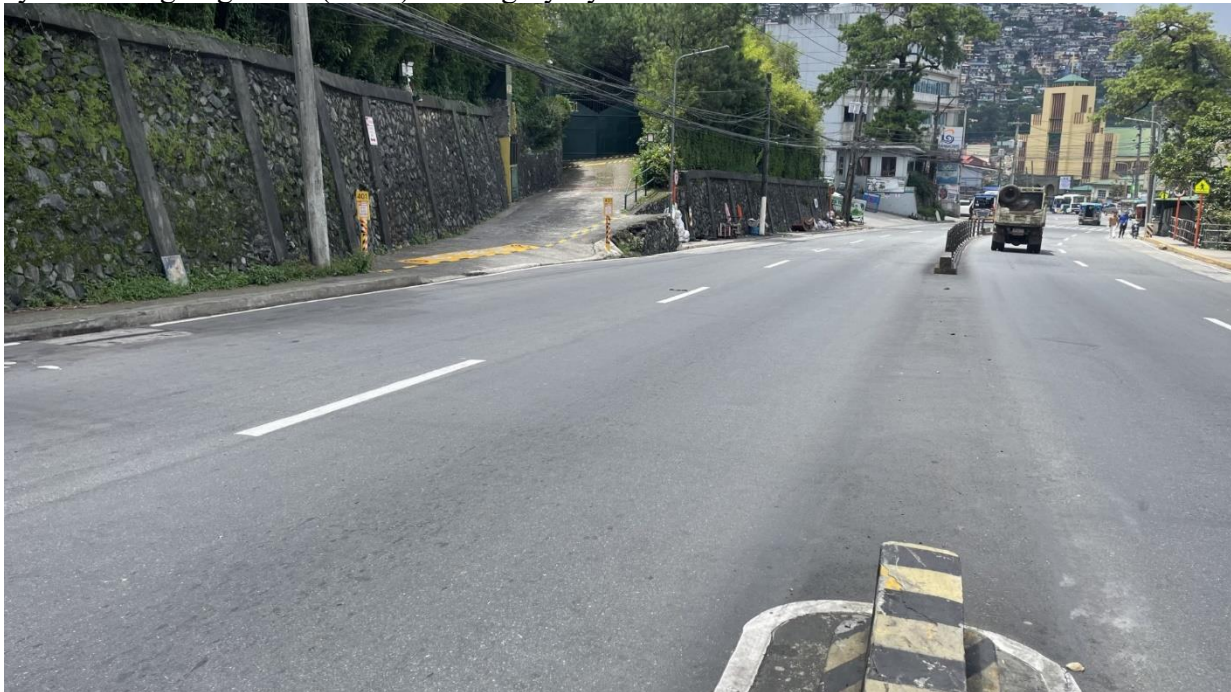
Driveway on left if going down (south) on Magsaysay Avenue.
